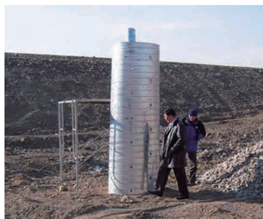
Pre installed Gas Removal Pipe
